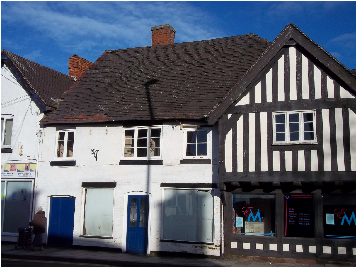
Photograph 1 showing 110 (left) and 111 Lichfield Street
